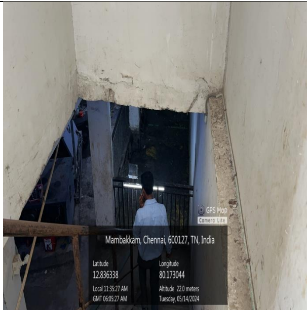
STP located at below ground level
